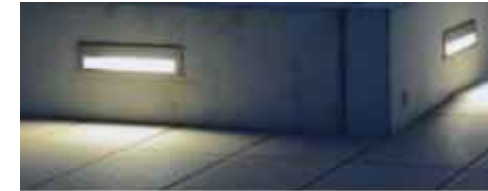
POSSIBLE WALL LIGHTS
